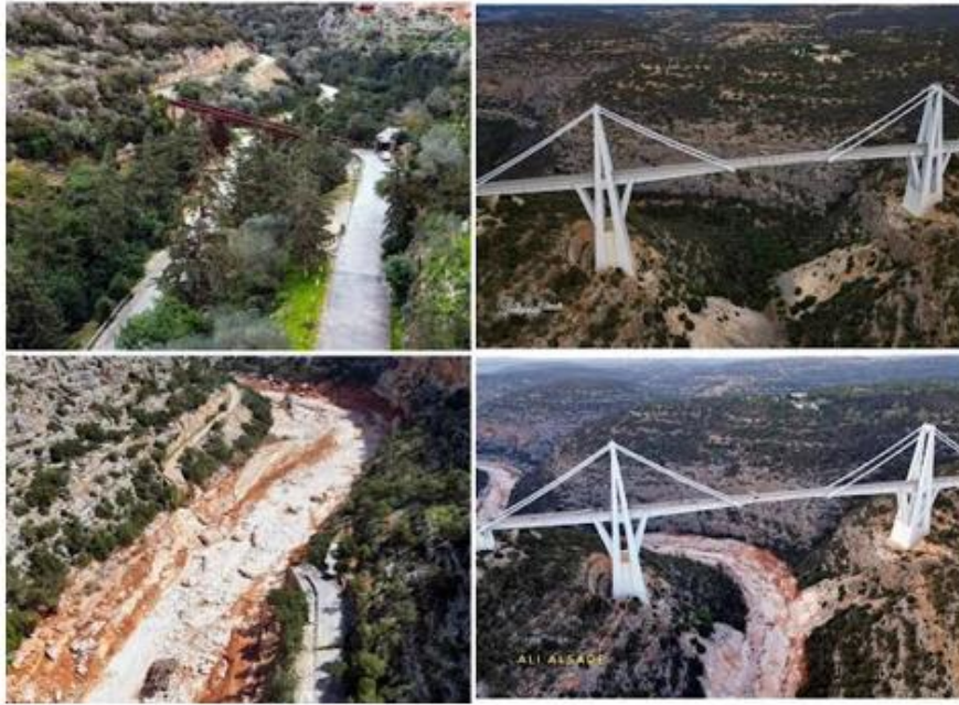
Figure 2. The catastrophic effect of Storm Daniel on Wadi Al kuf area from different locations. Left up, the wadi with the old bridge which established during Italian occupation before the flooding, and down, the devastation caused by the catastrophic flooding. Note the absence of the bridge, roads and vegetation. Right up the wadi new bridge. Note the differences between before flooding “up” and after flooding “down”. Photos were captured by the Libyan photographer Ali Al saadi (Al saadi, A., personal communication, October 10, 2023).
