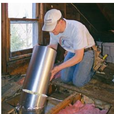
Figure (4.5) :A tubular skylight
