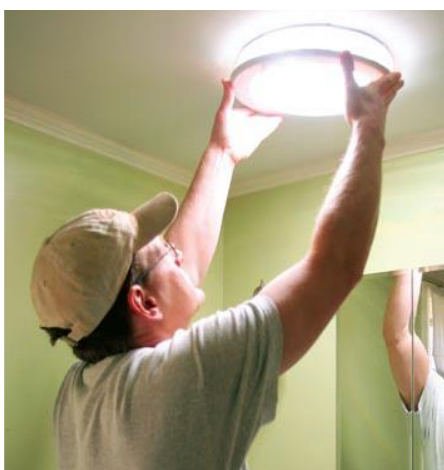
Figure (4.6) :From inside the house, a lighttube looks like a domed fixture
